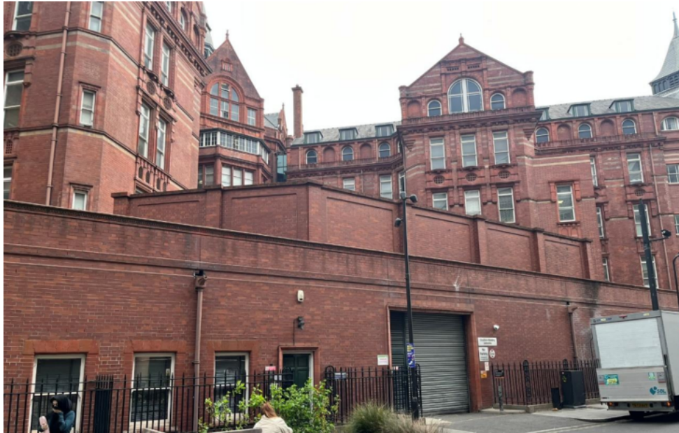
3. Photo of the rear of the building showing the existing brick plant screen
