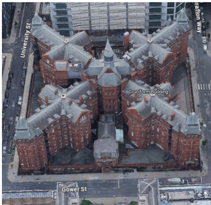
2. Aerial view of the building showing the front elevation
