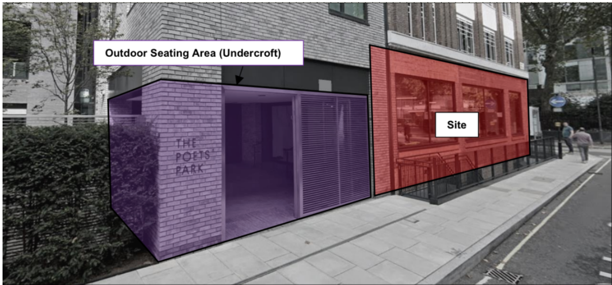
Photo 3 (above): View of the undercroft area with the ground floor unit beyond
