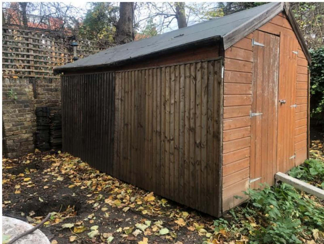
Figure 5. Existing rear shed (to be demolished)
