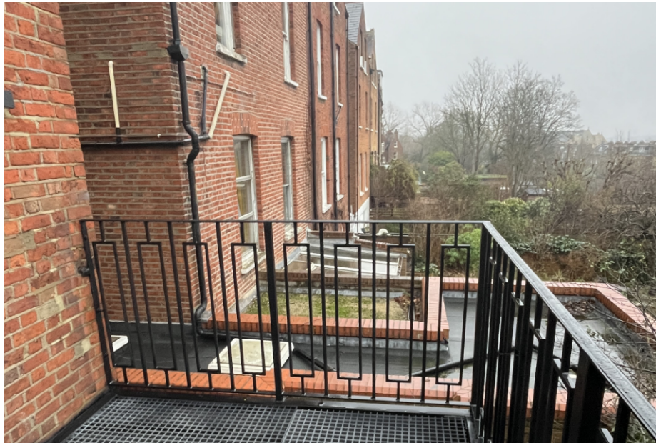
Photo 2 – view from balcony (as-built) at application site looking east
