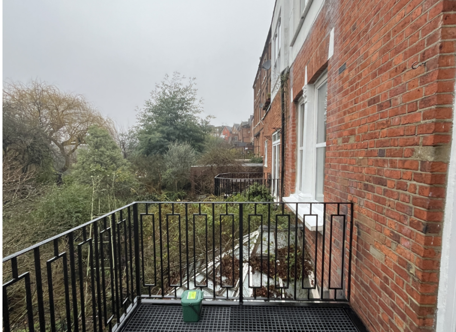
Photo 1 – view from balcony (as-built) at application site looking west
