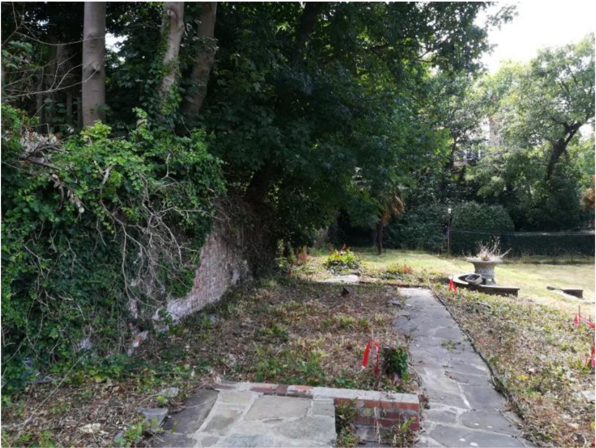
Figure 3 Looking southeast along the northeast flank of the site, showing the existing foundation element of the now-demolished outbuilding in the same general area as the proposed outbuilding (Source: submitted documents)
