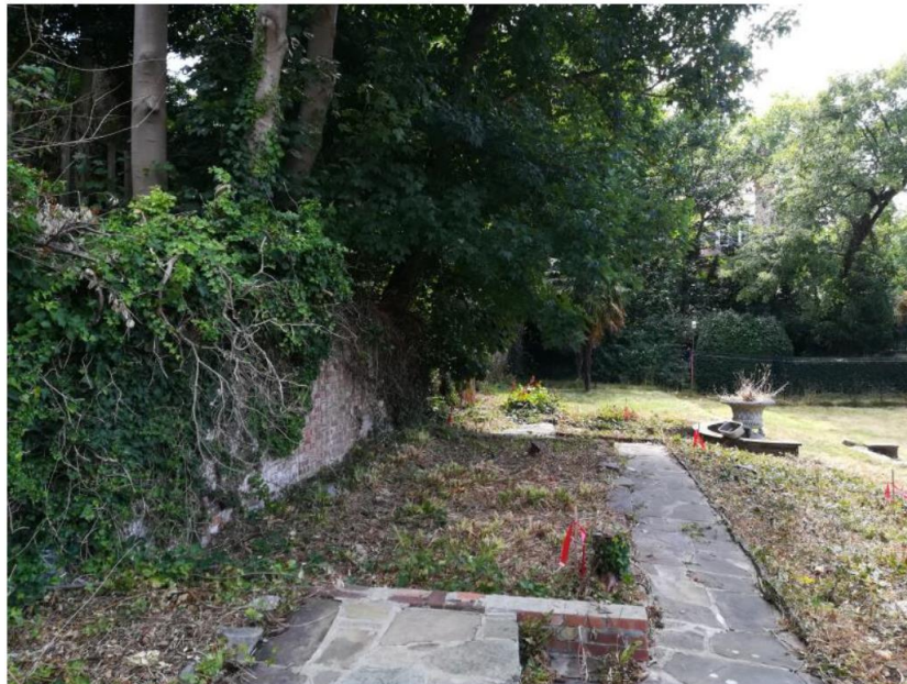
Figure 2 Remaining foundation element of the now-demolished outbuilding in the same general area as the proposed outbuilding
