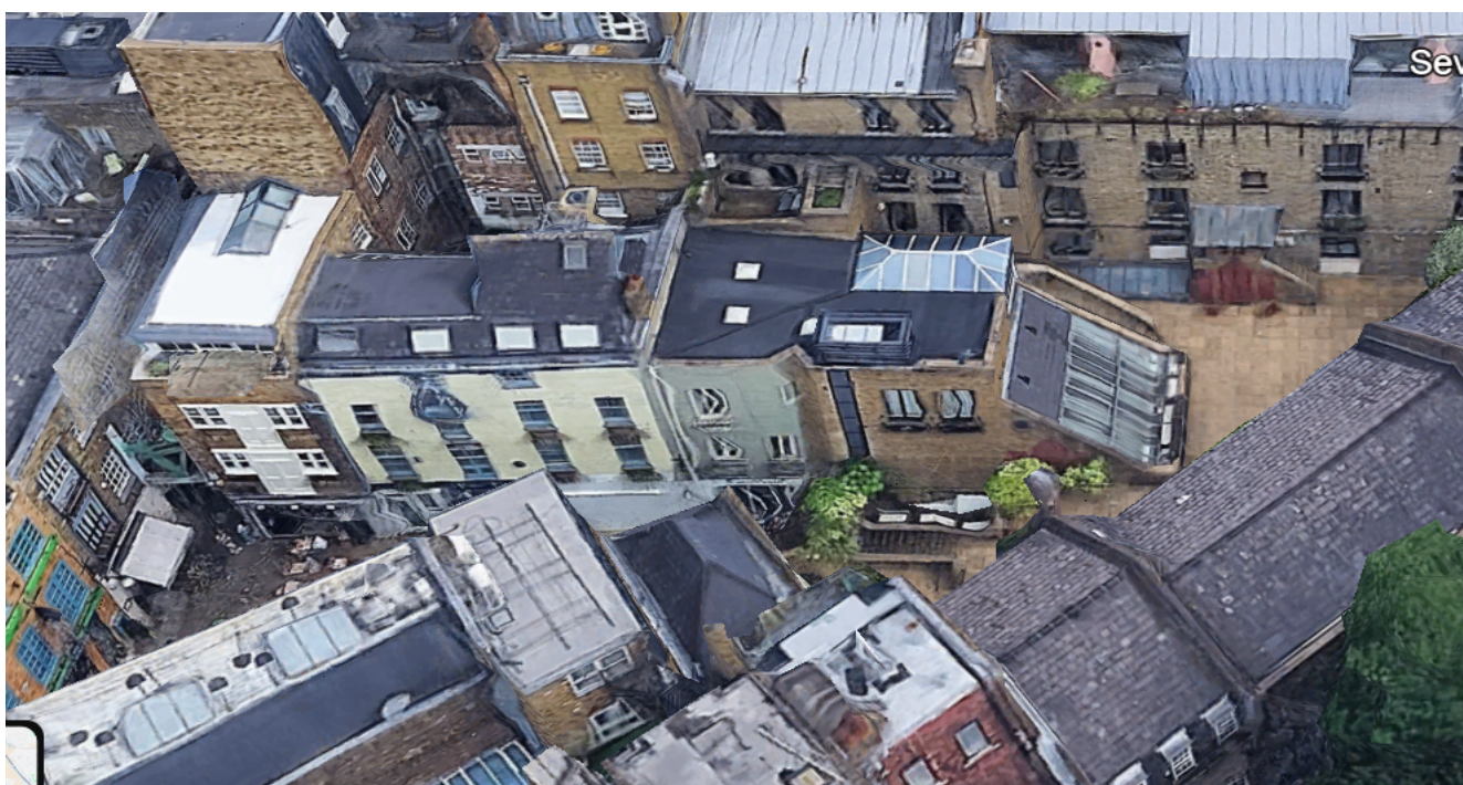
Figure 1. Showing the existing plant enclosure along the glass roof.
