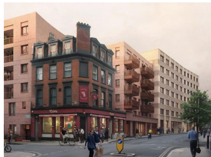
Jamestown Road Site Allocation C19. Planning permission granted 2025 and designed by Morris+Company, the scheme provides 187 student bedrooms, 27 affordable homes, and flexible commercial space, and is currently under construction.
