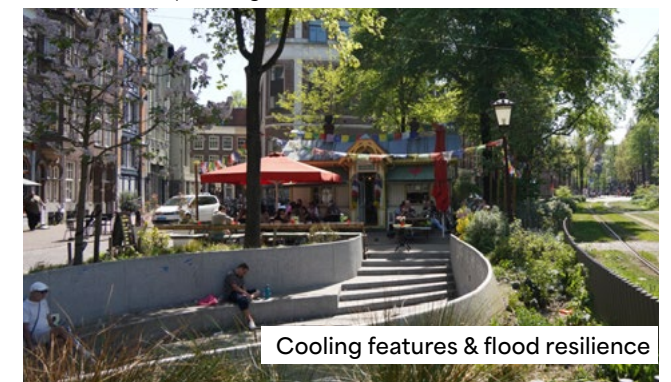
Het Blad is a water playground in Amsterdam. The pool's sides form seating when the pool is not filled and support a cooling space for play during hot weather. Planting and water attenuation is integrated into the design, further supporting climate resilience.
