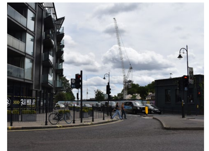
Parkway and Delancey Street Junction
