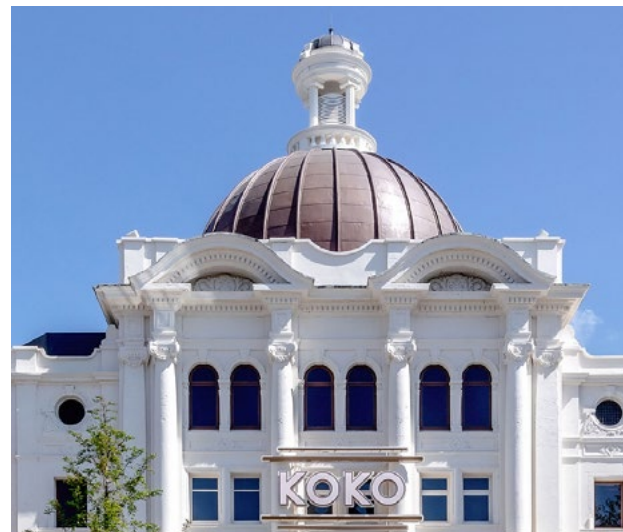
KOKO is an iconic live music venue in Mornington Crescent. Formerly the Camden Theatre, KOKO has recently undergone extensive restoration and reopened as one of London's last independent music venues, preserve its heritage and equipping it for a new future.
