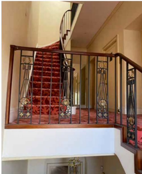
Stairs to Third floor
