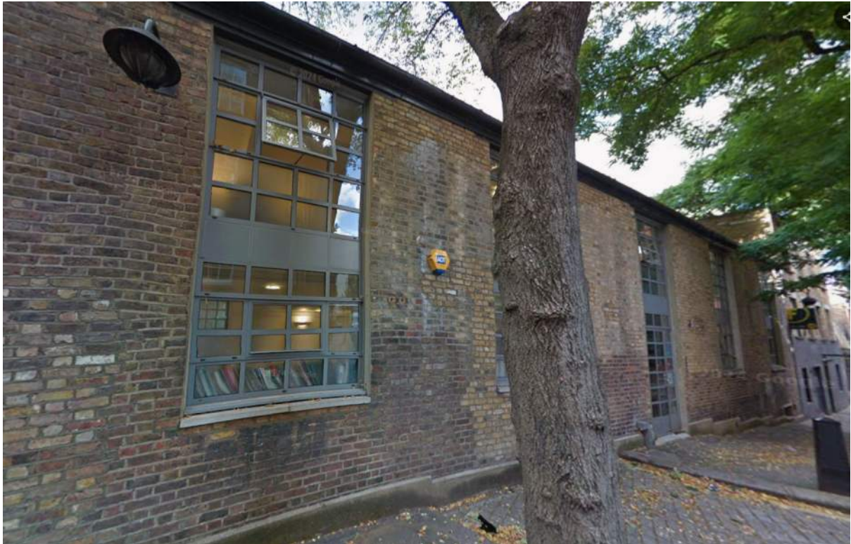
9. Google Street View image of the site from southwest corner (September 2018).
