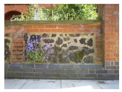
If you are rebuilding sections of boundary wall to match the existing, using matching bricks, matching mortar and matching the profile of the mortar pointing, this will not need planning permission. Unfortunately the over-zealous pointing on the left draws more attention to the mortar than the lava brick itself. This type of non-matching work is no longer permitted development, and repairs should be undertaken like-for-
