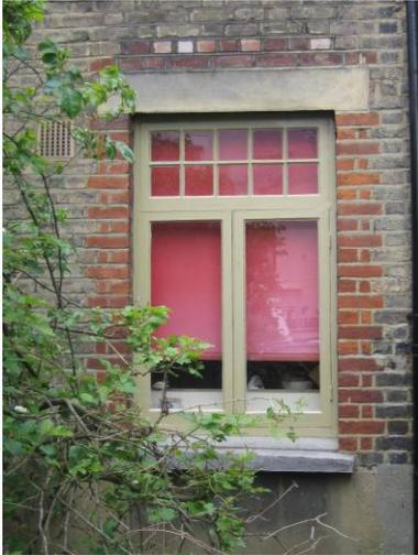
**1.4 Decorative glass** has an important ornamental role in addition to letting light into the building; it may be stained, etched held together with lead 'comes' or a combination of all three. It should always be retained and repaired and specialist advice should be sought (see: Key Contacts). *Its removal and replacement on front elevations (or side elevations where these front the street) needs planning permission and will be resisted.*
