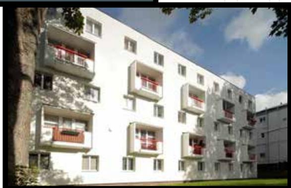
Kilburn Gate is a 1950s estate, owned by Camden Council, consisting of three blocks of 3 to 6 storey buildings. The 95 homes are occupied by a mix of tenants and leaseholders. The construction is of single skin non-cavity brickwork in English bond style. The thermal efficiency of the buildings was inadequate and did not meet the Decent Homes thermal performance standards.
