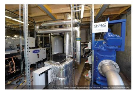
Figure 16 – Borden College Sharc Heat Exchanger and Filtration System
