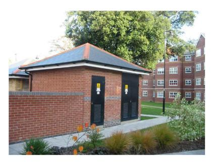
Figure 4 – UKPN standard brick substation enclosure
