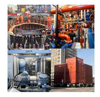
Figure 6 – Bunhill 2 energy centre GEA ammonia heat pump
