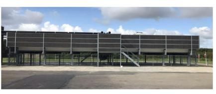
Figure 7 – 3MW air source heat exchanger with an acoustic screen
