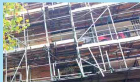
Scaffolding up at Radcliffe House at the Bourne Estate
