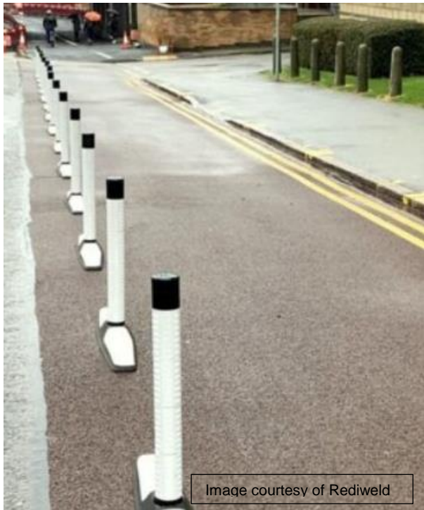
Image 4: 'Shared use bus boarder' (a raised section of cycle lane) placed at the bus stop, over which bus users have priority when boarding or alighting from a bus
