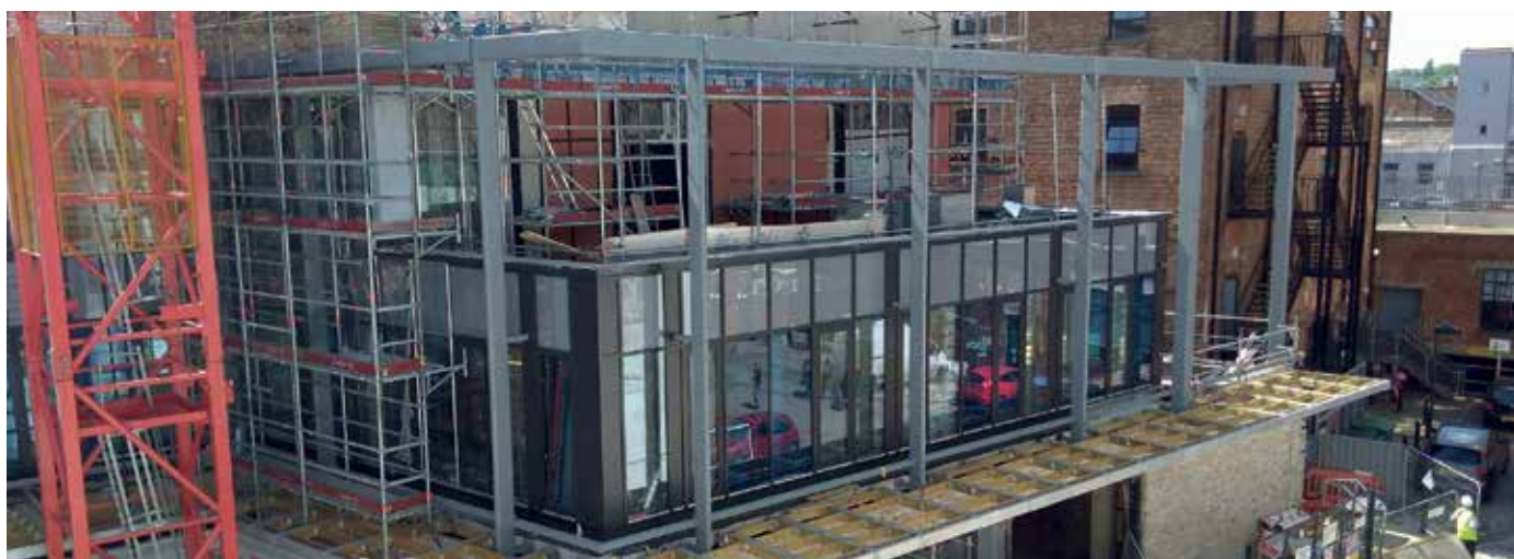
The Greenwood Centre under construction
