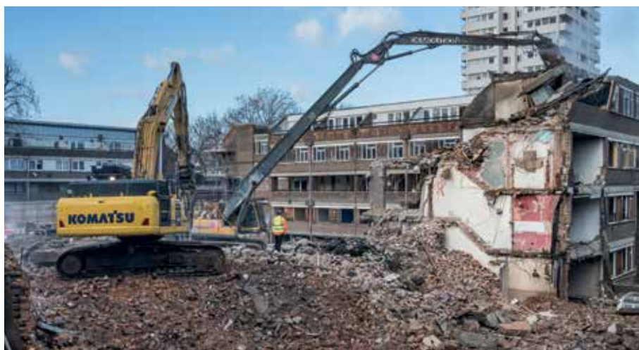
Demolition at Bacton Low Rise
