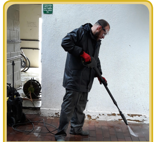
Caretaking teams jet washing communal areas in Durston
