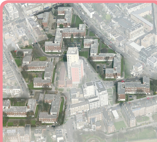
WEST KENTISH TOWN ESTATE BOUNDARY
