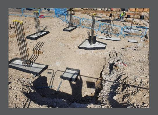
• Construction of pile caps to all blocks Aspen Court, Aspen Villas and Grafton Terrace (pile caps create a stable foundation and larger area to distribute the build load over)
