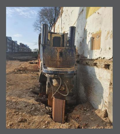
• Installation of sheet piling to existing gymnasium wall to retain the structures foundations
