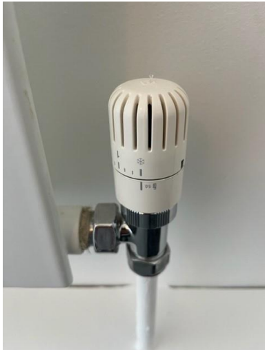
TRV turned to the off setting indicated by the frost symbol
