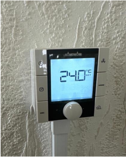
Trench heater thermostat turned on
