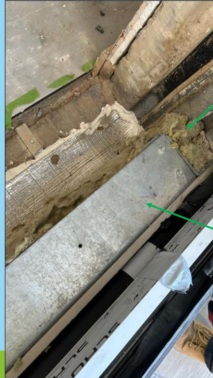
Metal cassette positioned into opening as base for the new window within the concrete structure of the building
